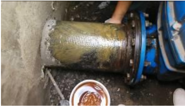
Photo 07 : View after apply STACprime
