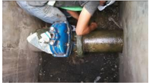
Photo 08 : Apply STACfill on flange area
