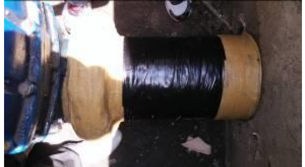
Photo 14 : View after apply STACguard
