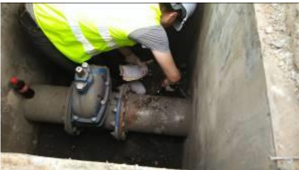
Photo 04 : Cleaning with hand tools
