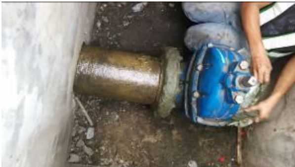
Photo 09 : View after apply STACfill
