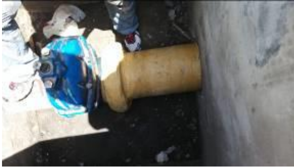
Photo 13 : View after apply STACwrap
