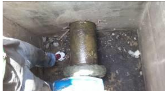
Photo 10 : View after apply STACfill
