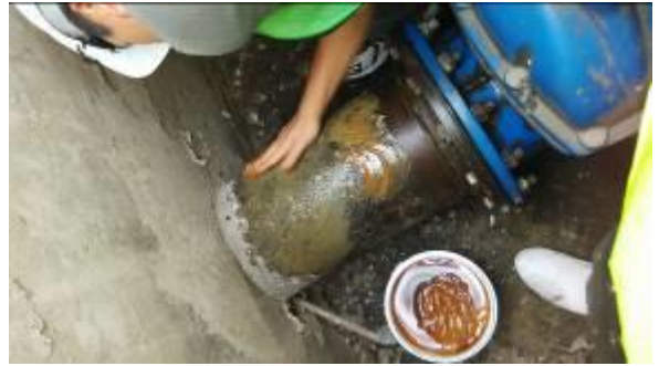
Photo 08 : Apply STACfill on flange area
