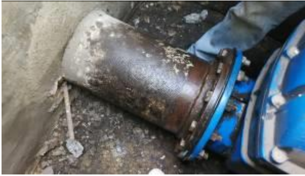
Photo 07 : View after apply STACprime
