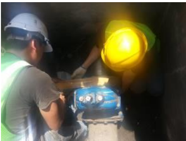
Photo 11 : View of apply STACwrap
